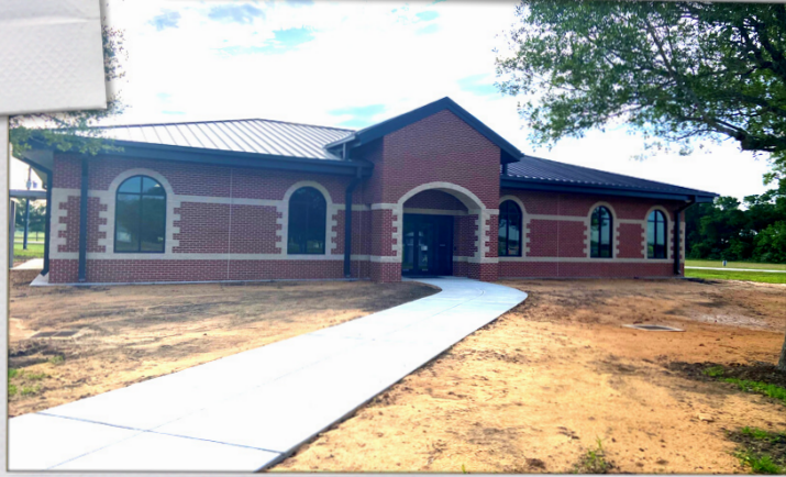
The new Rosenberg Development Corporation Building is nearing completion.
