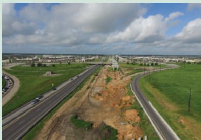
August 2016: I-69 southbound at FM 762 in the early stages of construction.
