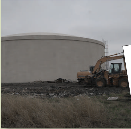
Water plant number 8, now under construction on A. Myers Road.
